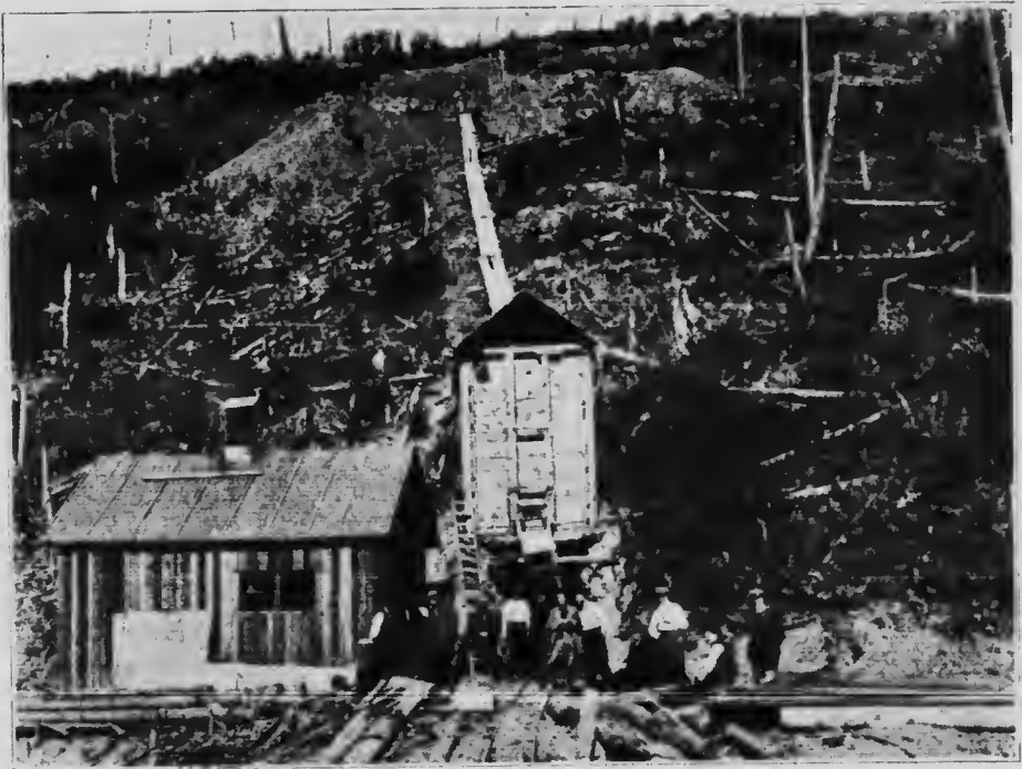
Showing Tunnel, Euton Mine, and Glory hole above.
