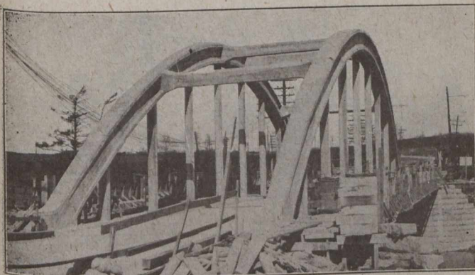
THE ETOBICOKE BRIDGE
