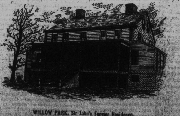
WILLOW PARK, Sir John's Former Residence.
