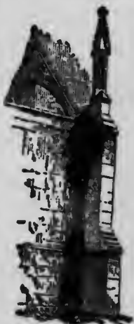
Buttress and Flying Buttress.
