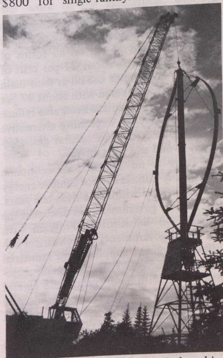
A 50-kilowatt vertical axis wind turbine being erected on Vancouver Island.
