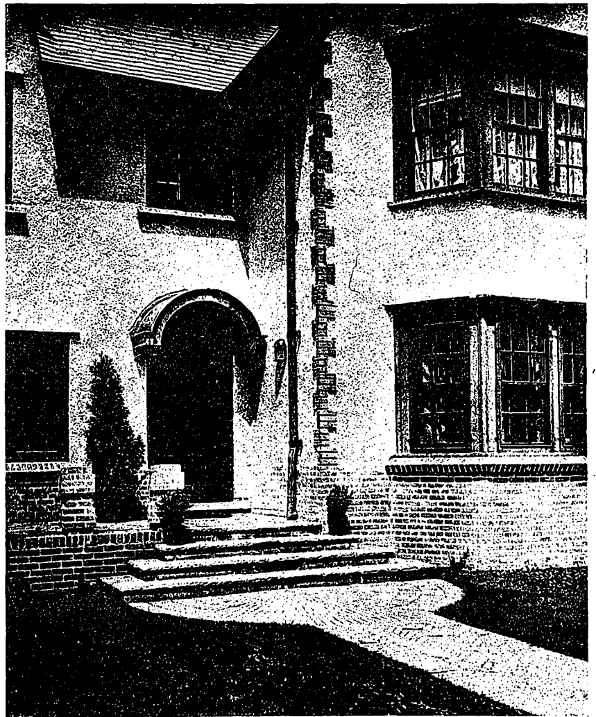
DETAIL OF MAIN ENTRANCE, HOUSE NO. 1.
