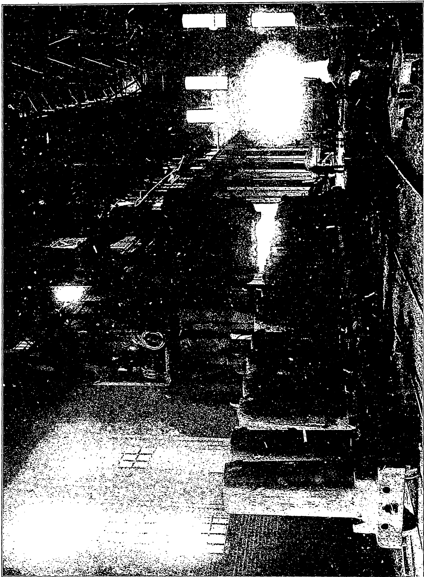
Interior of Furnace Plant Dominion Iron and Steel Company at Sydney, Cape Breton, showing Kettle discharging Molten Pig Iron into ingot cars for transmission to Converters.
