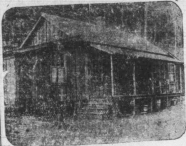
A 'good school,' but bare and uninviting. Shows lack of interest in surroundings.
