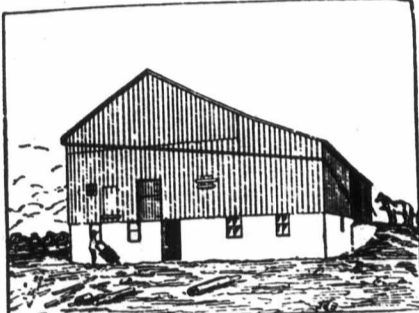
Barn of Benjamin Pile, Parkhill, Ont. Size of Walls, 50 x 81 x 10 feet high. BUILT WITH THOROLD CEMENT IN 1898.
