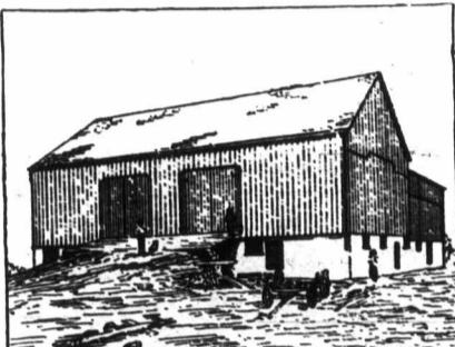
Barn of Allan McMane, Atwood, Ont. Size of Walls, 84 x 100 x 9 feet high. BUILT WITH THOROLD CEMENT IN 1898.
