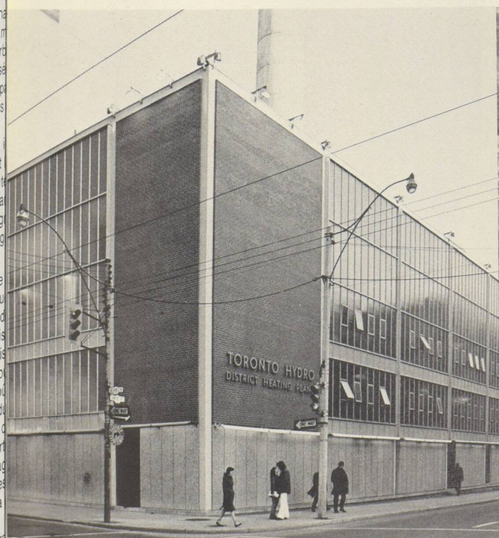
District heating plant operated by Toronto Hydro. • Centrale de chauffage urbain de l'Hydro Ontario.
