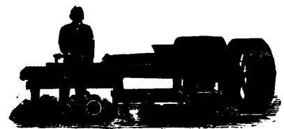
Kell's Patent Brick and Tile Machine.
