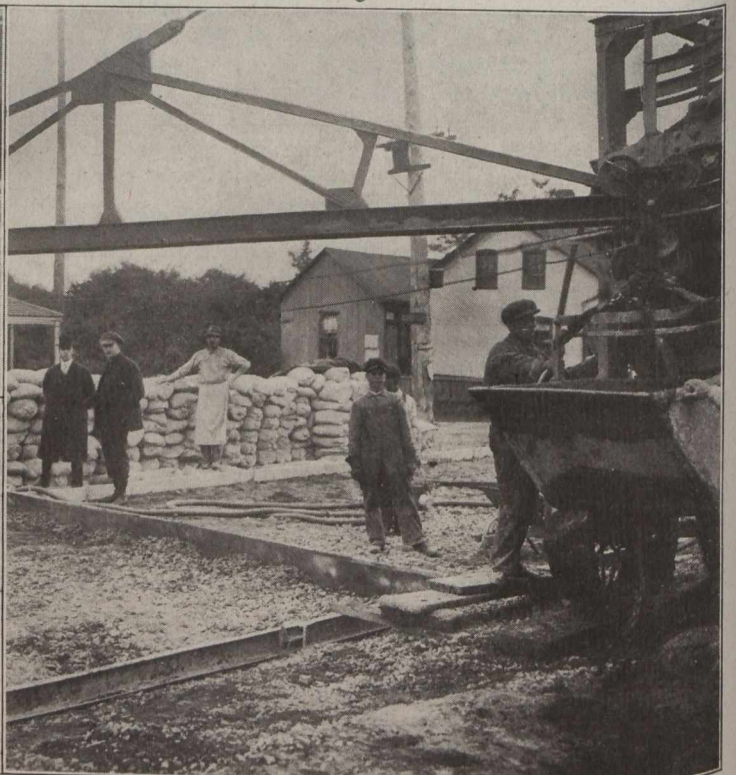
Steel Forms and Form Set-up to Support Felt Expansion Joint.
