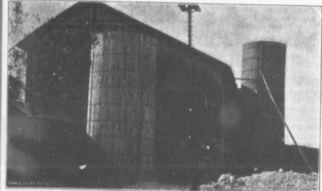
Two Low-Cost Silos—Ours Used for Summer Feeding
