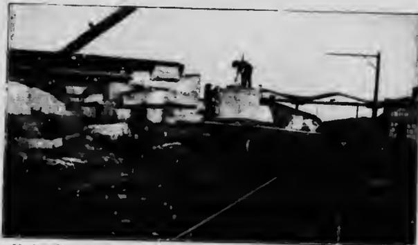
*Unloading stone brought from a quarry, where it was cut into blocks, placed on flat cars, and shipped to its destination.*
