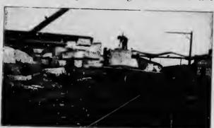
Unloading stone brought from a quarry, where it was cut into blocks, y aced on flat cars, and shipped to its destination.
