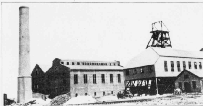
POWER HOUSE AND BANKHEAD, ALLAN SHAFTS, ACADIA COAL CO.
