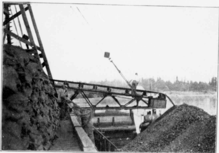
LOADING SCOW BY BELT-CONVEYER, PACIFIC COAST COAL CO., BOAT HARBOUR, V.I.
