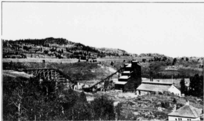
WASHERY AND POWER PLANT, LEITCH COLLIERIES, PASSBURG, ALTA.
