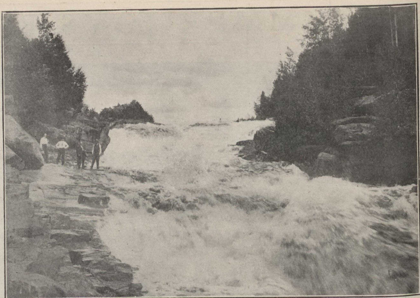
An Artificial River used as a Log Chute, from a small lake near Lake Temiskaming.
