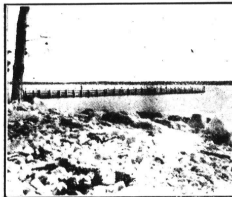
Breakwater and boulders
