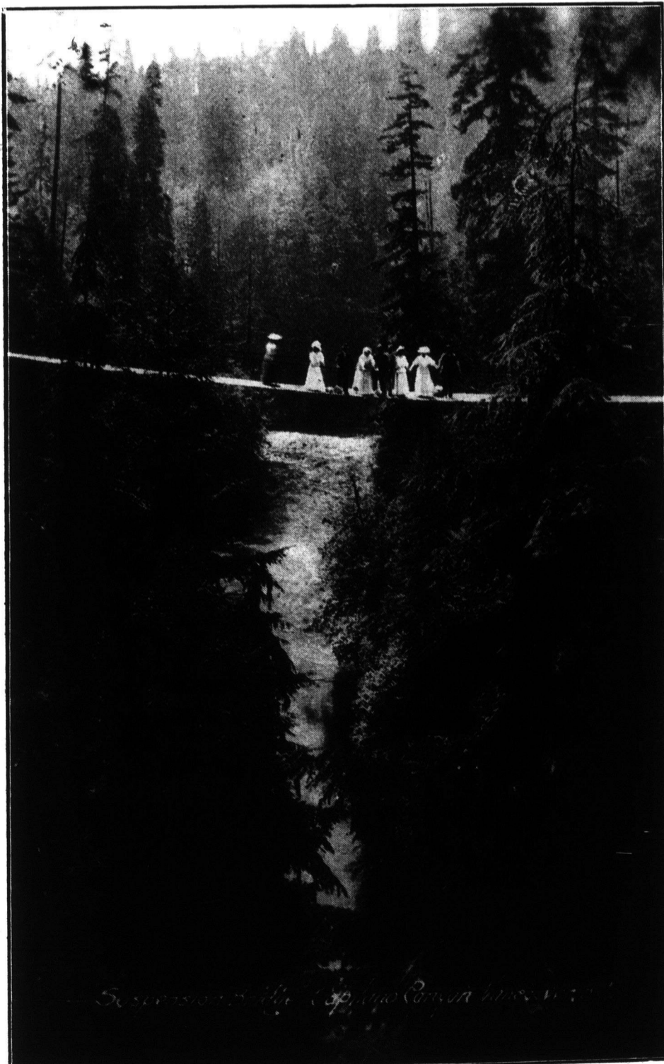
Suspension Bridge, Capilano Canyon, Vancouver, B.C.
