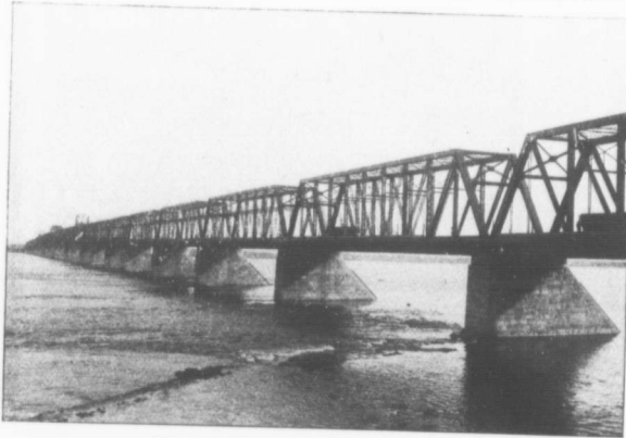
Victoria Jubilee Bridge — re-constructed 1897.
