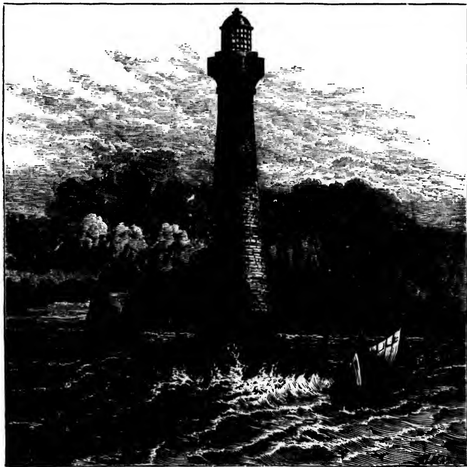
THE SKERRYVORE LIGHTHOUSE.
