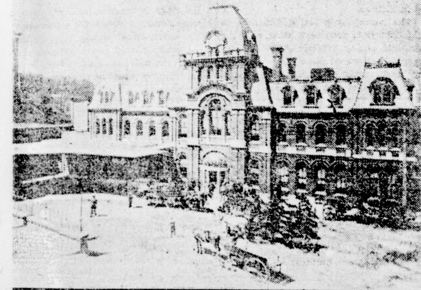
(Reported to have collapsed.)
