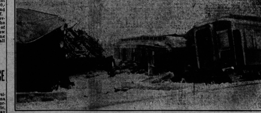
ANOTHER AULAC WRECK SCENE. The Demolished Cars as they Appeared from across the Right of Way. Several of the Coaches are only fit for Kindling Wood.
