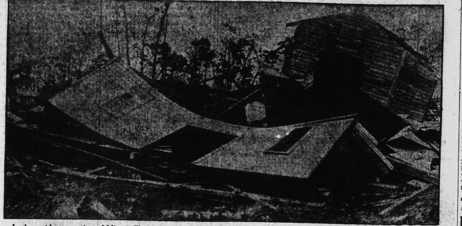
In the residence section of Miami, Fla.—since the storm. Homes were bowled over like houses built of cards. Here is a flattened out section of street, with a frame cottage knocked into a pancake design and a portion of the barn piled on top as if in antic fire. The scene is typical of miles of street in "the wonder city of the tropics."
