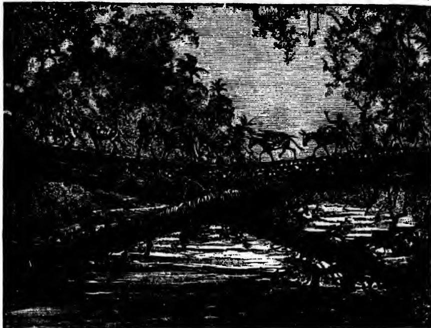
EXPEDITION CROSSING A TEMPORARY BRIDGE.
