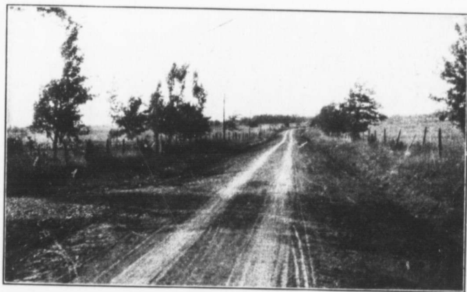
Permanent Stone Road as Built under the County System.
