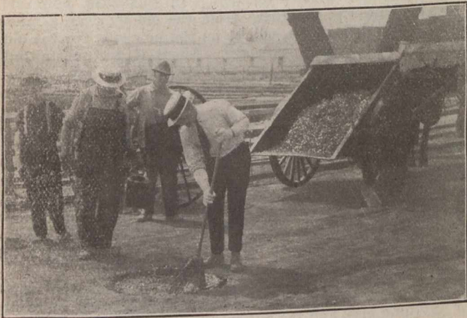
FIG. 4—PAINTING BOTTOM AND SIDES OF HOLE
