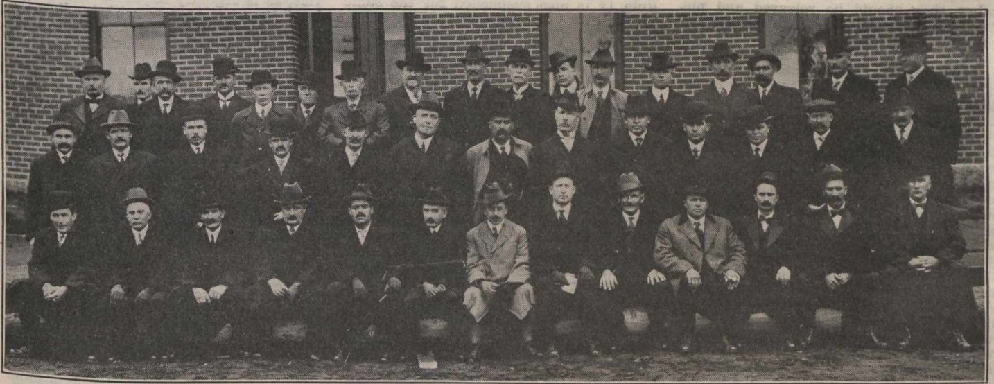
C.P.R. Track Maintenance Inspection Party at Farnham, Que.
