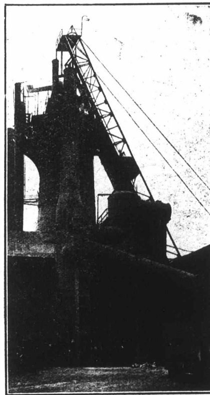
Exterior View of Blast Furnace Showing Pipes for Conveying Waste Gases to Stoves. Dust Separator in Foreground.
