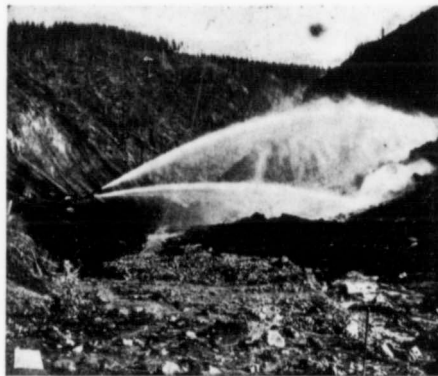
Two 8-inch streams opening up Pit No. 2 at S. Fork Mine, Cariboo.
