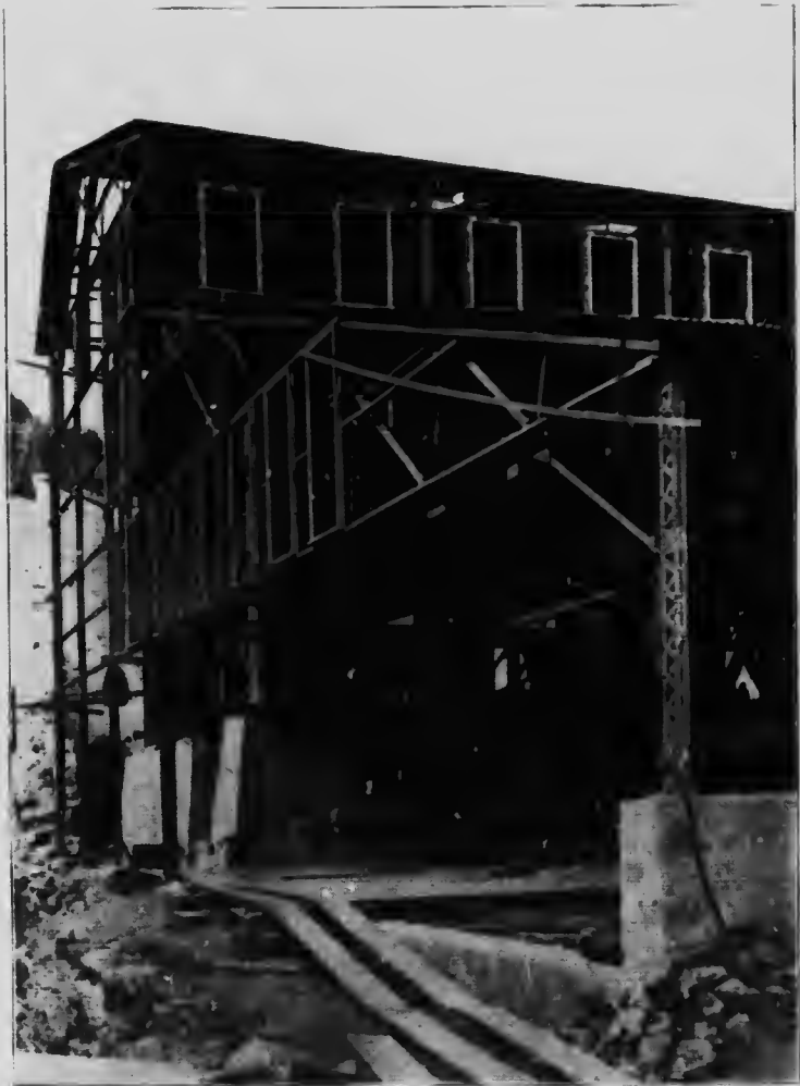
STEEL ORE-BINS AND BATTERY FOUNDATIONS OF THE BUSTOS MILL
