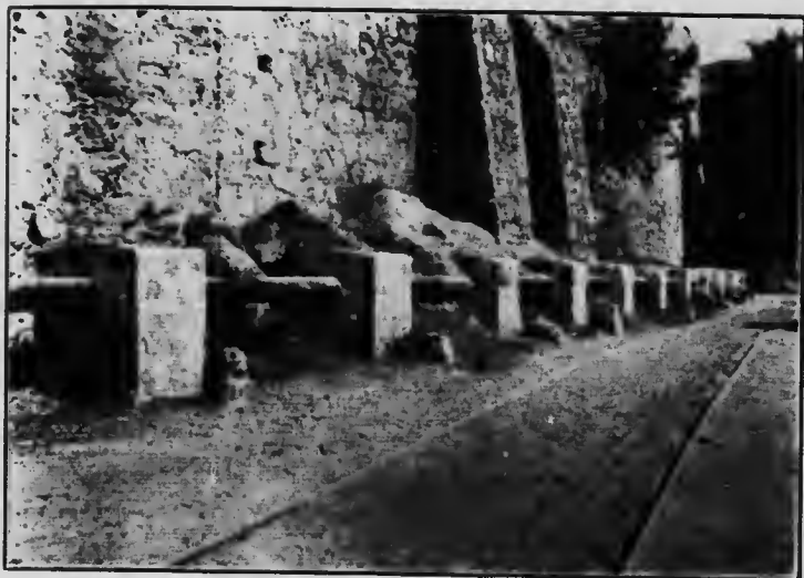
PIPE-LINE FOR CONVEYING TAILING
