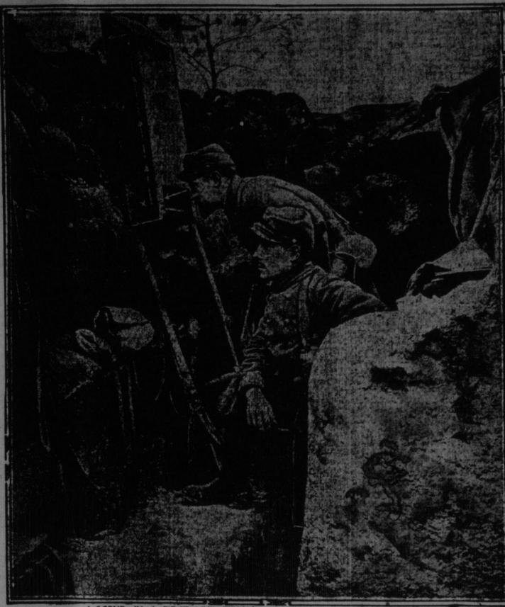
A SCENE IN A FRONT LINE TRENCH SHOWING THE LAND PERISCOPE IN USE. THE MOST NOTICEABLE OBJECT IN THE TRENCH IS, OF COURSE, THE PERISCOPE, WHICH IS USED FOR OBSERVING THE MOVEMENTS OF THE ENEMY WITHOUT EXPOSING THE OBSERVER TO UNNECESSARY RISKS. THE PERISCOPE CONSISTS, IN THE MAIN, OF TWO MIRRORS, THE ANGLES OF WHICH ARE SO ADJUSTED THAT THE OBSERVER CAN WATCH THE GROUND IMMEDIATELY IN FRONT OF THE TRENCH WITHOUT HIMSELF BEING SEEN.
