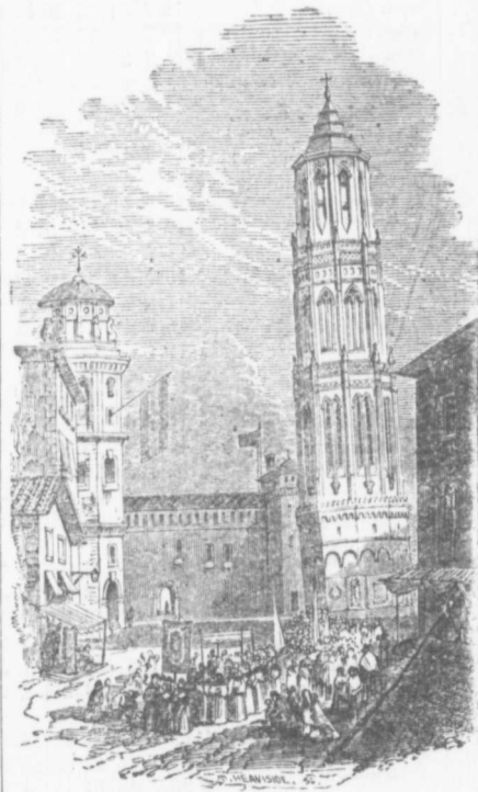
LEANING TOWER, SARAGOSSA.
