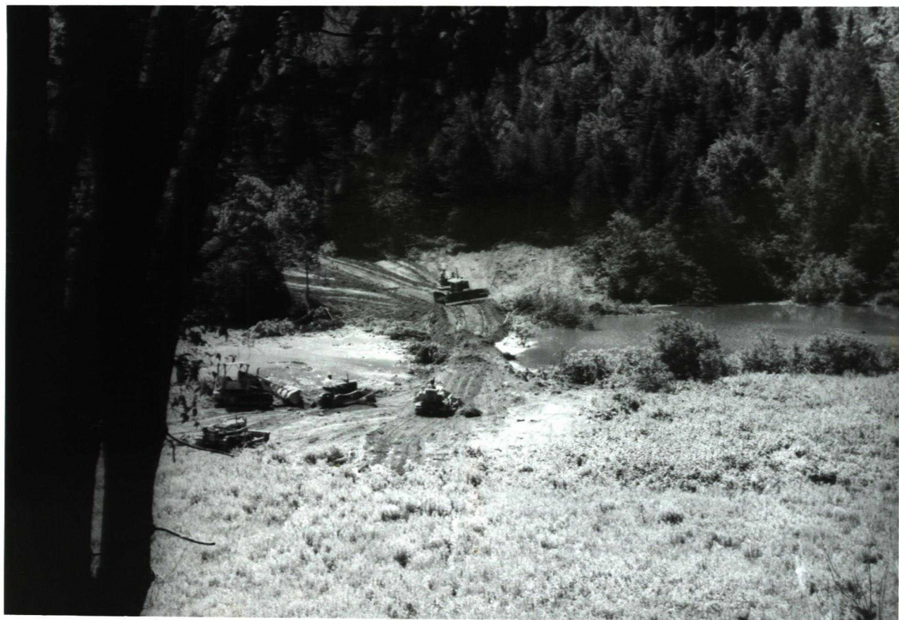
Dam under construction on the International Boundary. July 9, 1968
