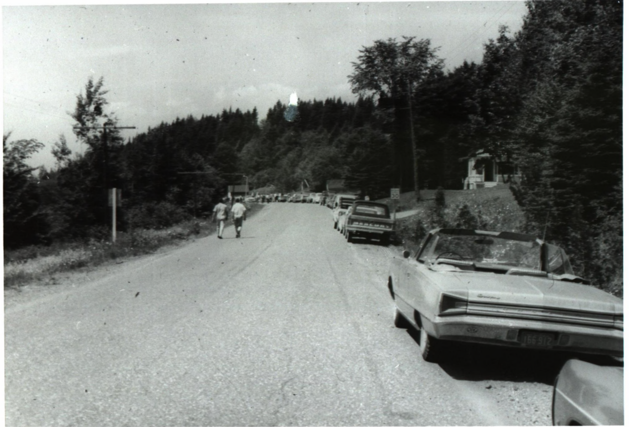
Cars and crowds assembled on the highway to view the dam construction. July 9, 1968.
