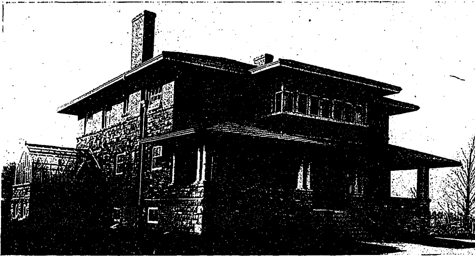
RESIDENCE OF M. G. HENNIGER, CONTRACTOR, SMITH'S FALLS.
