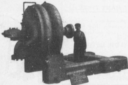
Worthington 2 Stage Turbine Pump for the Winnipeg Water Works, Capacity 5,000,000 per 24 hours.
