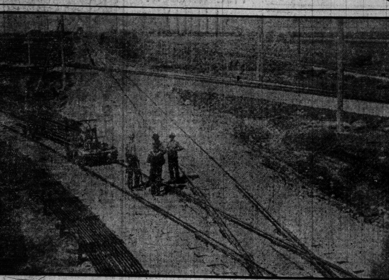
A UNIQUE MEETING POINT: Four Transcontinental Railways, the Grand Trunk Pacific, Canadian Pacific, Canadian Northern and Great Northern meet at Portage La Prairie. The pipes shown on left contain the signal wires, all controlled from one signal tower.
