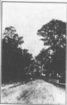
Cut No. 85 Building Protecting Walls Around Trees.
