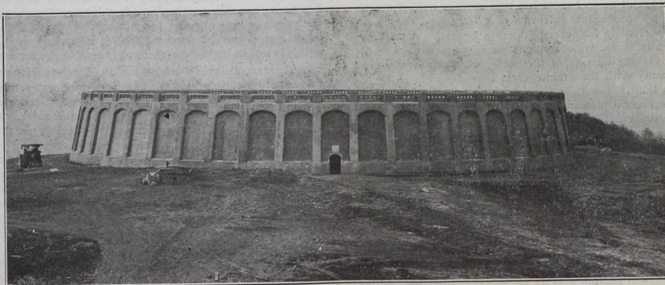
Fig. 4.—Nearing Completion, Exterior View.
