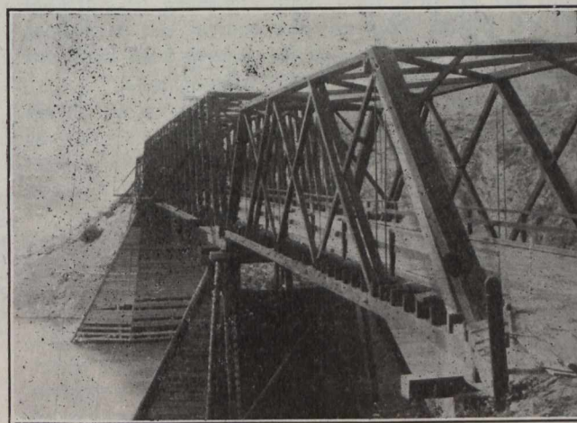
Fig. 1.—Bridge at Lytton, B.C., Which is Being Replaced.
