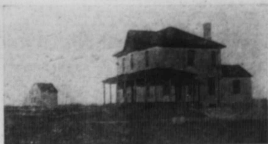
Superintendent's Residence on Nursery Station at Indian Head, 1905
