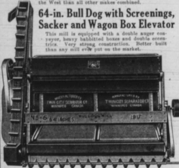
Note the Double Auger Conveyor; one for Screenings, one for Seed Grain.
