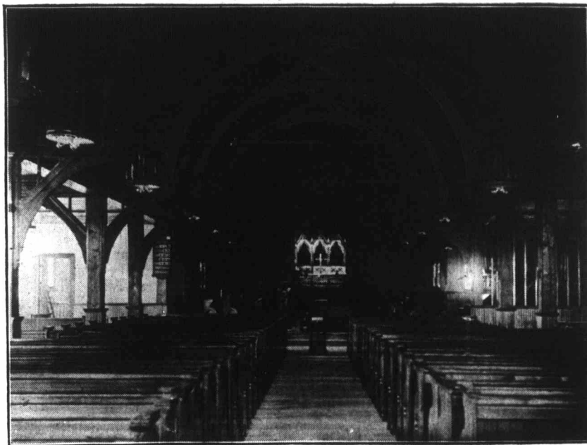
St. Matthews', Ottawa. Interior as Enlarged and Beautified, September 1908. Seating Capacity, 900.
