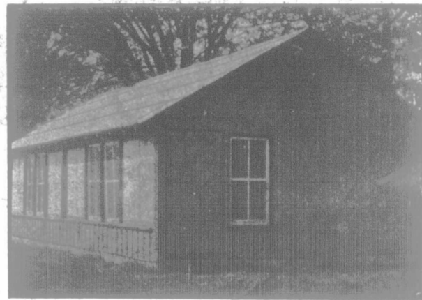
House with double-pitch roof and straw loft to absorb moisture.
