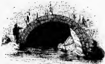
Cloaca Maxima (the great sewer) at Rome.
