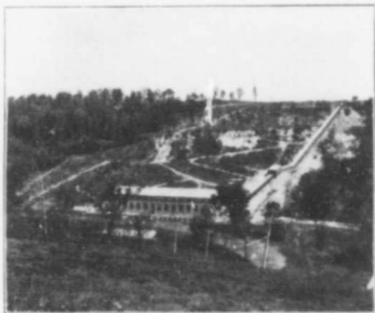
The Power House at DeCew Falls.
