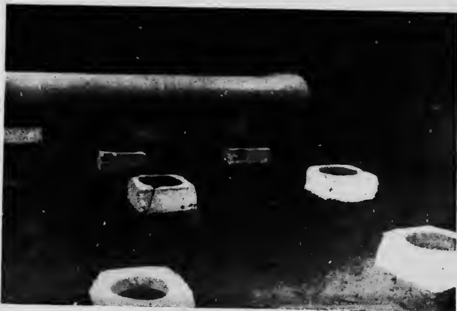
PLATE V.—Interior view of an underground system of ventilation designed by S. McKenna. This system is especially valuable in curing heavy bodied tobacco. The cold air enters the tile at A (Plate 5) coming up into the barn at B directly under the flue and is heated before coming in contact with the tobacco. Each tile shown in Plate 5 leads to a different opening in the floor, and, as there are eight of these lines of tile on each of the two sides of the barn, there are sixteen of the openings shown in Plate 6 in the floor of the barn.
