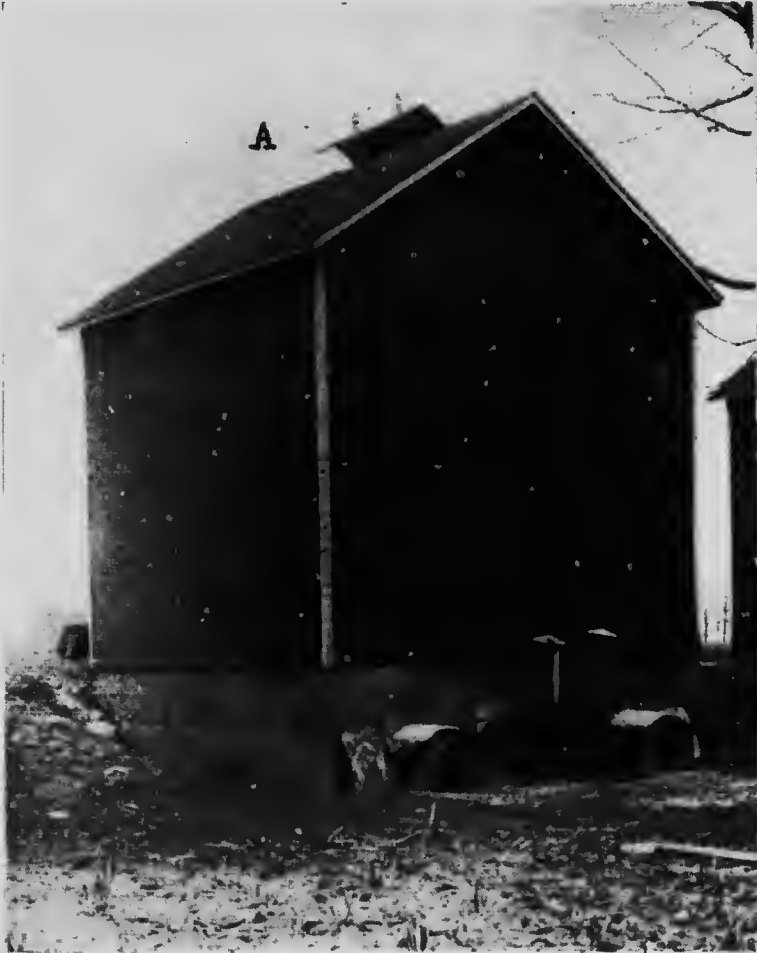
PLATE VII.—Exterior view of curing barn, showing fire-places and top ventilation.
