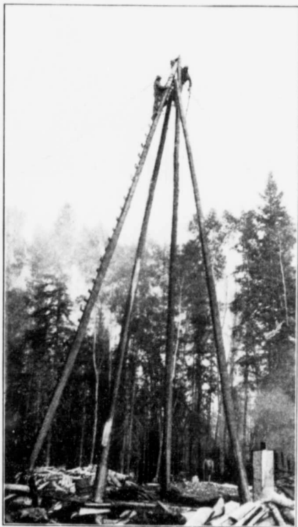
Derrick at No. 2 well in course of erection, Athabaska Oils, Ltd., 9 miles below Fort McKay, Alberta.
