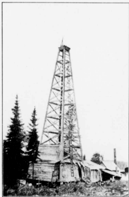
No. 1 rig, Athabaska Oils, Ltd., 9 miles north of Fort McKay, Alberta.
