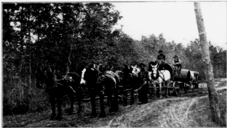
Hauling boiler from Edmonton to Athabaska, Alberta, 1911.
