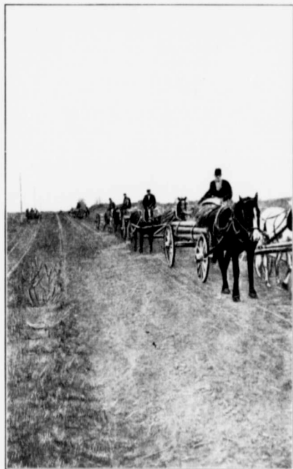
Hauling casing from Edmonton to Athabaska, Alberta, 1911.
