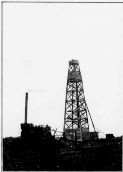
Dry hole at Taber, Alberta, showing traction engine used in drilling.
