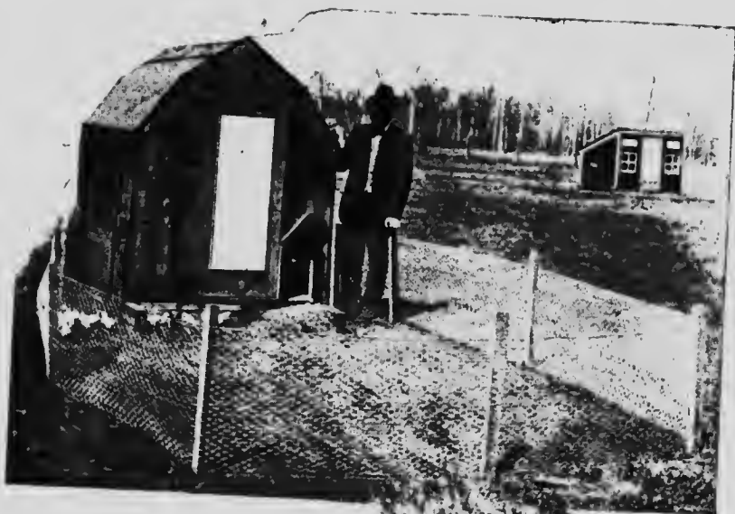
Fig. 7—This portable colony house for rearing chickens is made out of two piano boxes, with the backs taken out and placed back to back, on 3x6 inch runners...The illustration shows the method of yarding chicks until they are two weeks old at the College.
