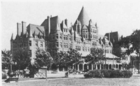
PLACE VIGER HOTEL AND PASSENGER STATION, MONTREAL
