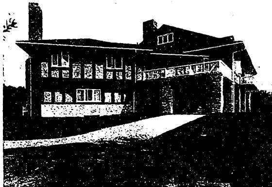
VIEW SHOWING LEFT WING, COUNTRY HOME OF MR. JAMES RYRIE. BURKE AND HORWOOD, ARCHITECTS.
