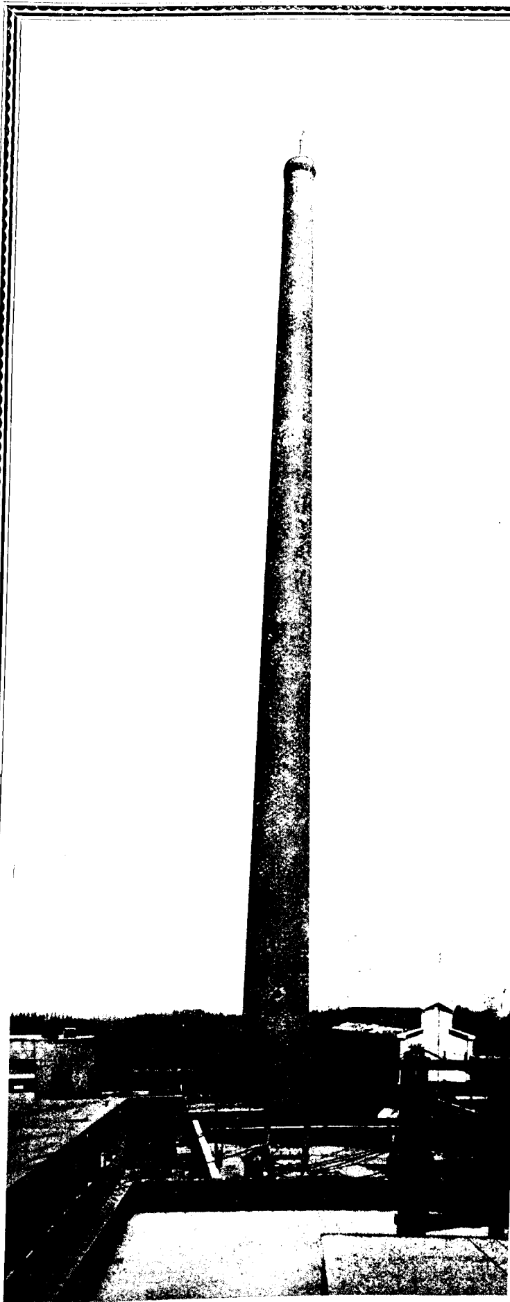
Chimney Built by Us at Rochester, N. Y., for the Eastman Kodak Co.—366 Feet High.
