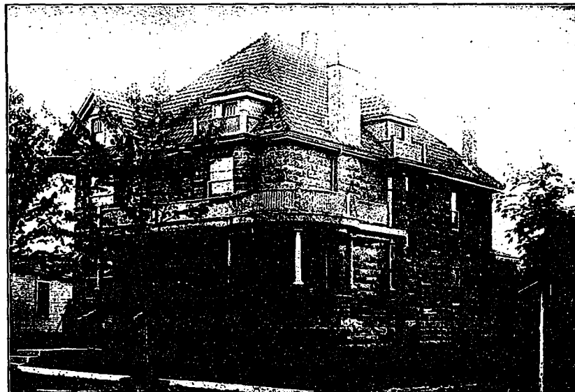
A $2,400 RESIDENCE. ALL THE BLOCKS USED WERE MADE ON THE CONCRETE BLOCK MACHINE MANUFACTURED BY THE LONDON CONCRETE MACHINERY COMPANY, LONDON, ONT.
