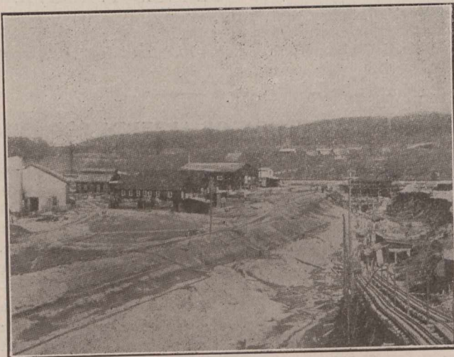
Fig. 1.—General View at the West Portal, Showing Plant and Tunnel Entrance as Seen at Present.
