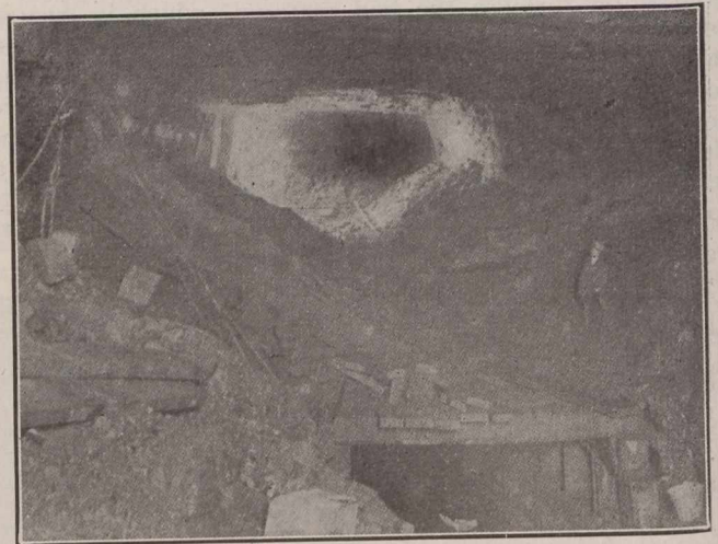
Fig. 5.—Break-up Excavation, Showing Bottom Heading With Jumbo Timbers.
