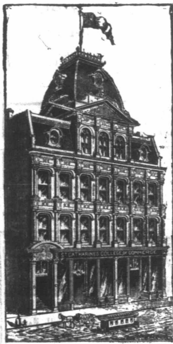
THE COLLEGE occupies the ground floor and first story of this superb structure. It is unquestionably the finest, most thoroughly modern school of business and shorthand training in Canada, and also the cheapest. Circulars free.
